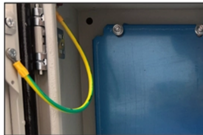
Grounding screw More aesthetically pleasing and safer
